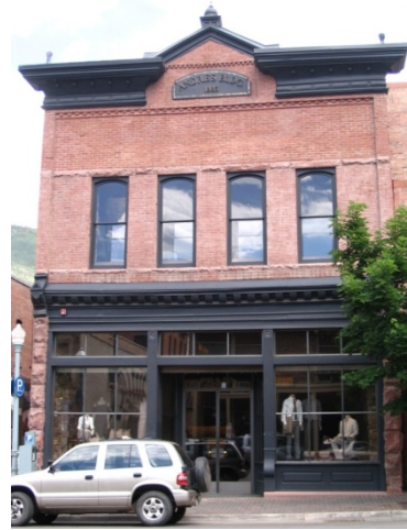
Original storefront columns exposed to view again. Windows reconstructed based on historic photographs.
