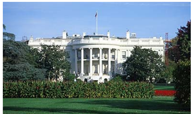
A portico, added in 1824, transformed the White House into a Neo-Classical building.
